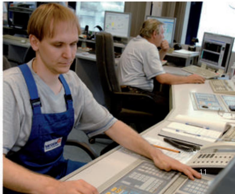
All the units are remotely monitored from the Control Center in Budapest.
