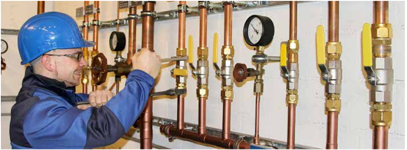
Stefan Fuchs, a technician at Messer in Switzerland, installing the piping for supplying medical gases in a hospital.
