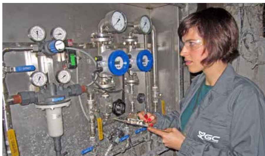
A Gomà-Camps employee notes down readings from the CO 2 control module.
