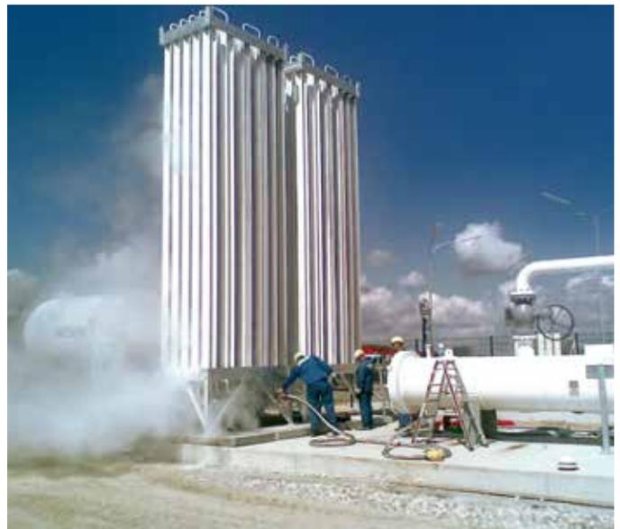
A 70-kilometre section of high-pressure natural gas pipeline was purged with 2,000 cubic metres of nitrogen per hour.
