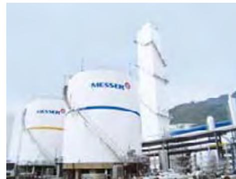
The new air separation units have a total capacity of 35,000 standard cubic metres per hour.
