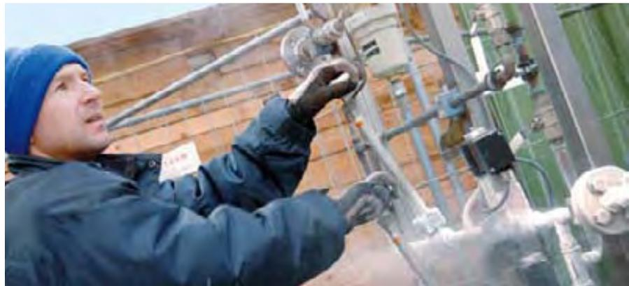
The volume of liquid nitrogen can be controlled precisely during cement cooling.
